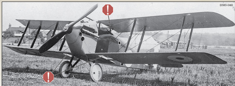
^ Sopwith Dolphin 2nd prototype in its initial form with radiators mounted in the top wings. Note the cutouts in the bottom wing intended to improve downward visibility which in practice turned out to be completely useless.
